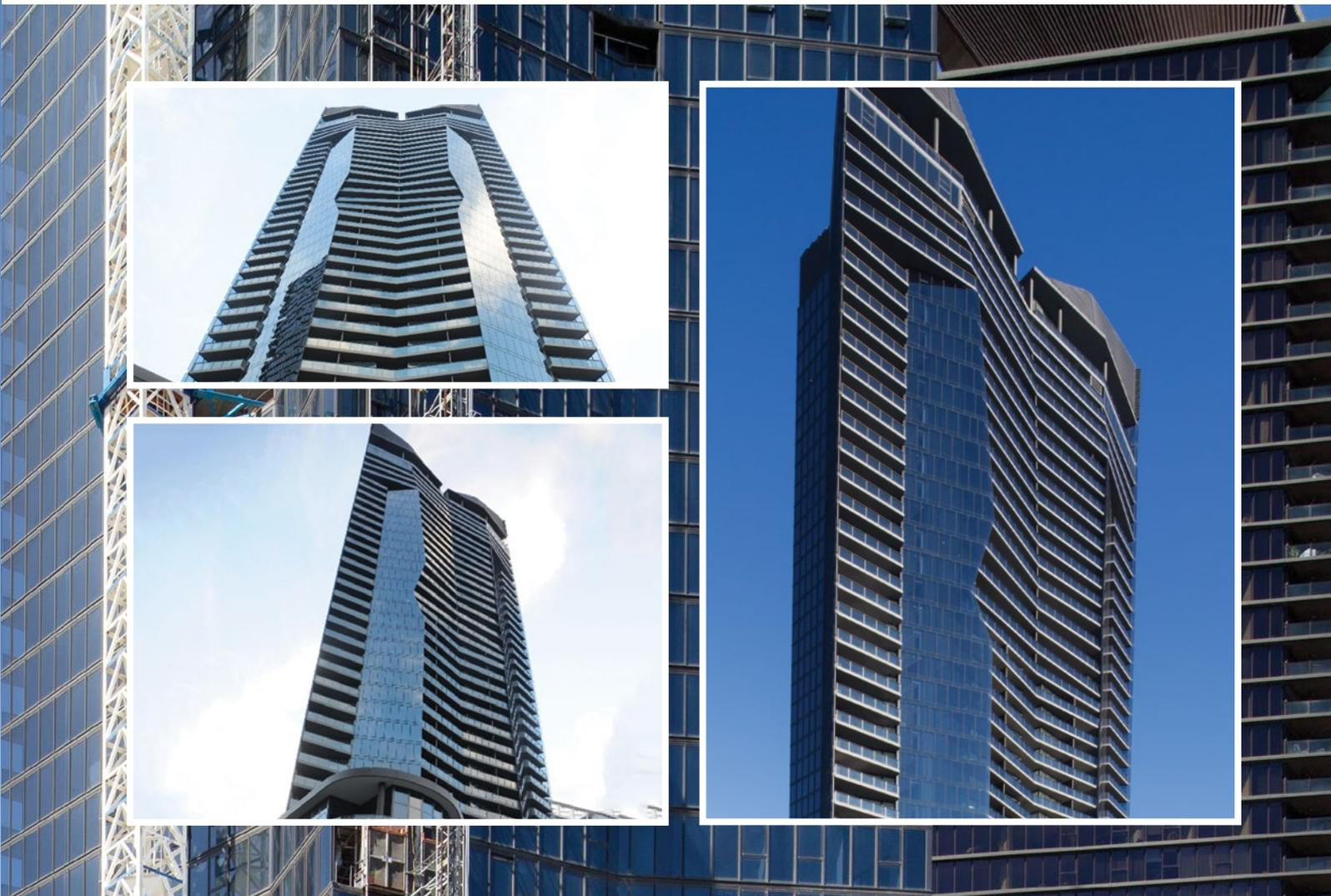
**Micos is leading the way in Australia as a premium supplier of Glass and Aluminium façade solutions.** The team at Micos provided products and services for the Array Docklands, Melbourne. The works included the design (that contained a fully bespoke system development specifically for this project), engineering, fabrication, delivery and installation of all the external fully enclosed glazed façade elements.
